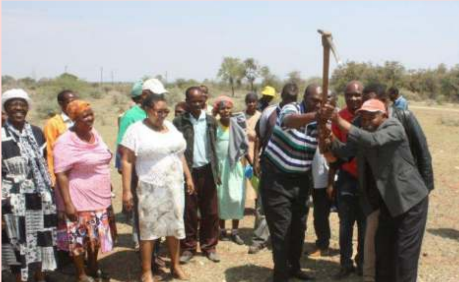
Mayor Selamolela and the community leaders break ground marking the official commencement of the construction of Kgatlu Creche.
